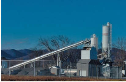
New Boxley Concrete plant on Aerial Way Drive
