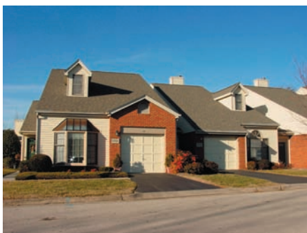
Existing house in Windsor Place Planned Unit Development
