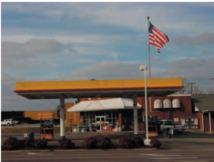
Existing gas station at Brandon and Edgewood
