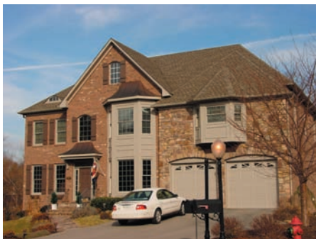
Existing house on Hidden Oak Road
