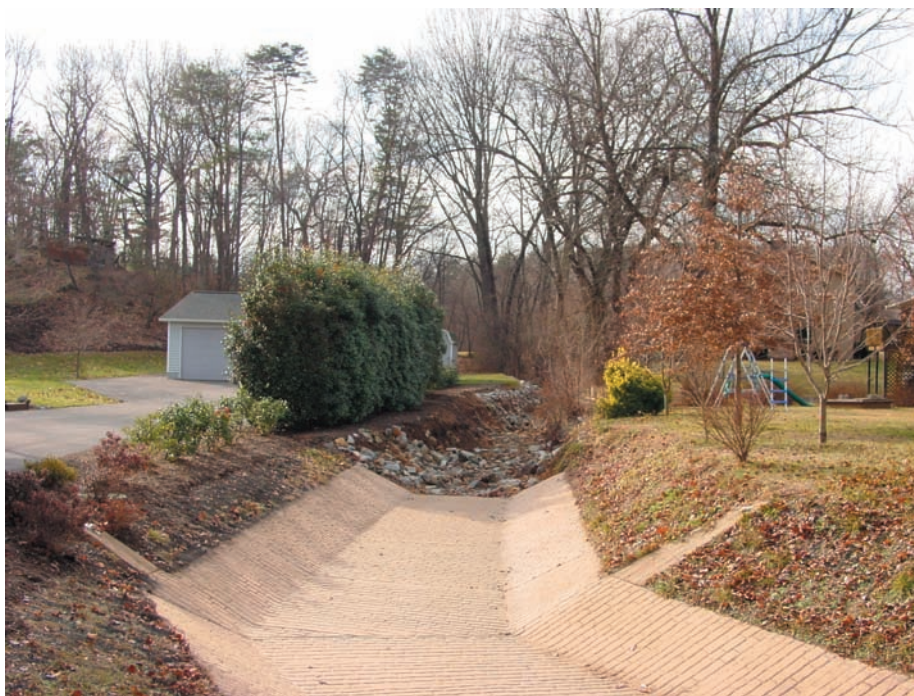
Erosion and Sediment Control measures implemented along Mudlick Creek
